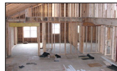
An interior view of the new CIB building.
