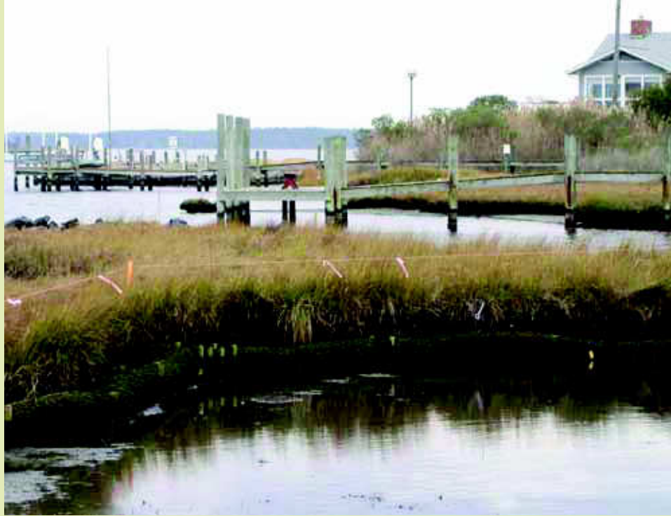
The staked coir fiber logs (usually made entirely from natural coconut fibers) reduce wave energy, provide an area for plants to grow, trap sediment, and degrade after several years.
